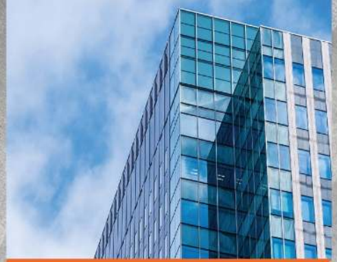
Cephe Sistemleri / Facade Installations
