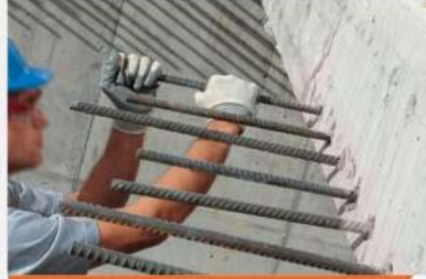
Filiz Ekimi Anchorage Installation
