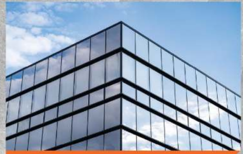
Cephe Sistemleri / Facade Installations
