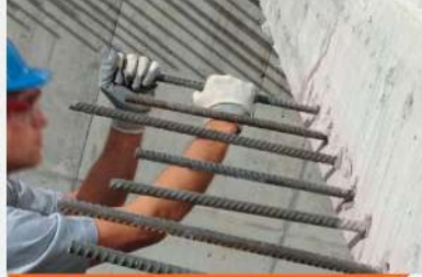
Filiz Ekimi Anchorage Installation
